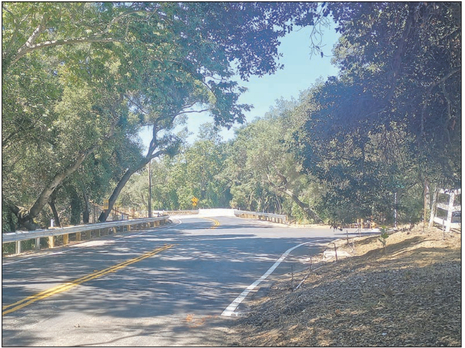
After a year-long project between Caltrans, the Department of Public Works and Rainbow Water Supply, a completed Live Oak Park Bridge Replacement is ready for cars at the intersection of Live Oak Park Road and Gum Tree Lane. The previous 25 foot long triple arch culvert bridge was replaced by a concrete slab bridge. Village News/Jenna Ortiz photo
